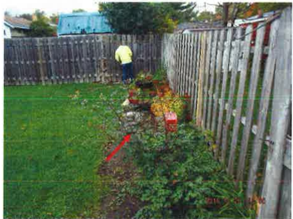
#4: Approximate PR Location Looking North from 1011 South Summit; Fence R&R-E
