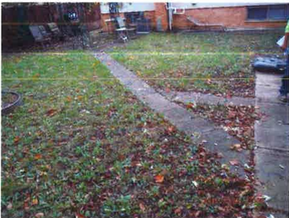
#5: Remove and replace (R&R) Concrete Patio Stones as needed (838 Grant's Backyard)
