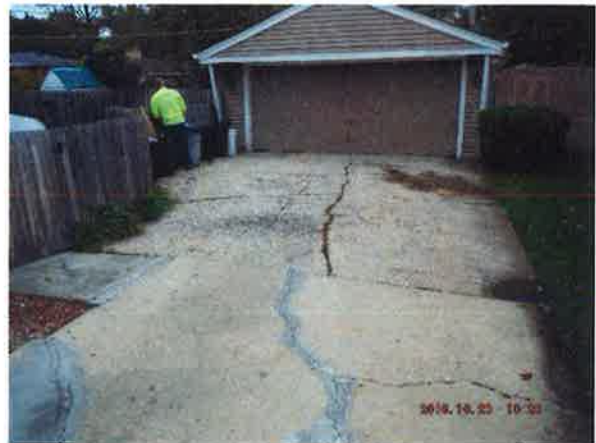
#2: End of Driveway (Possible Access Route); Fence R&R-E
