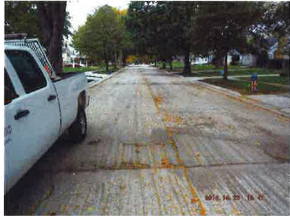
#2: Road Surface removed; Concrete Subbase – looking West
