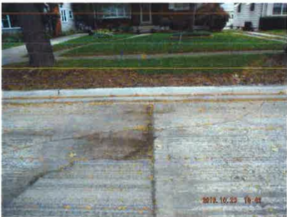
#5: Approximate Location of the existing lateral service connection – Looking North
