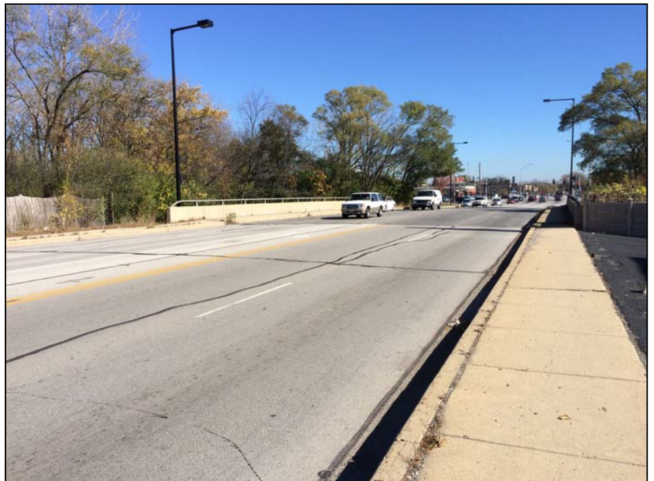
Photograph of St. Charles Road Bridge deck, looking east.
