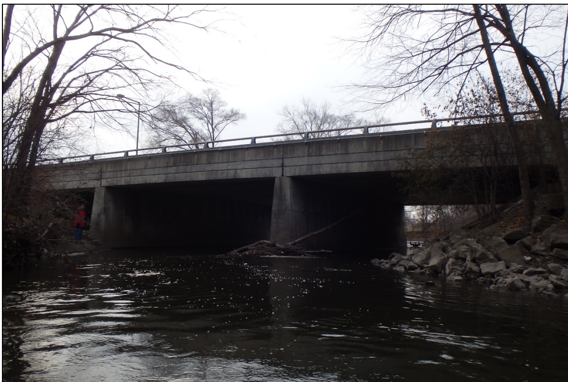
Photograph 2: Overall View of Bridge No. 022-6950, Looking Southeast.
