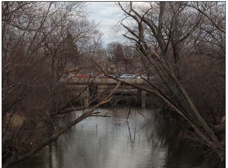
Photograph of the Route 83 Bridge downstream of the Pedestrian Bridge.
