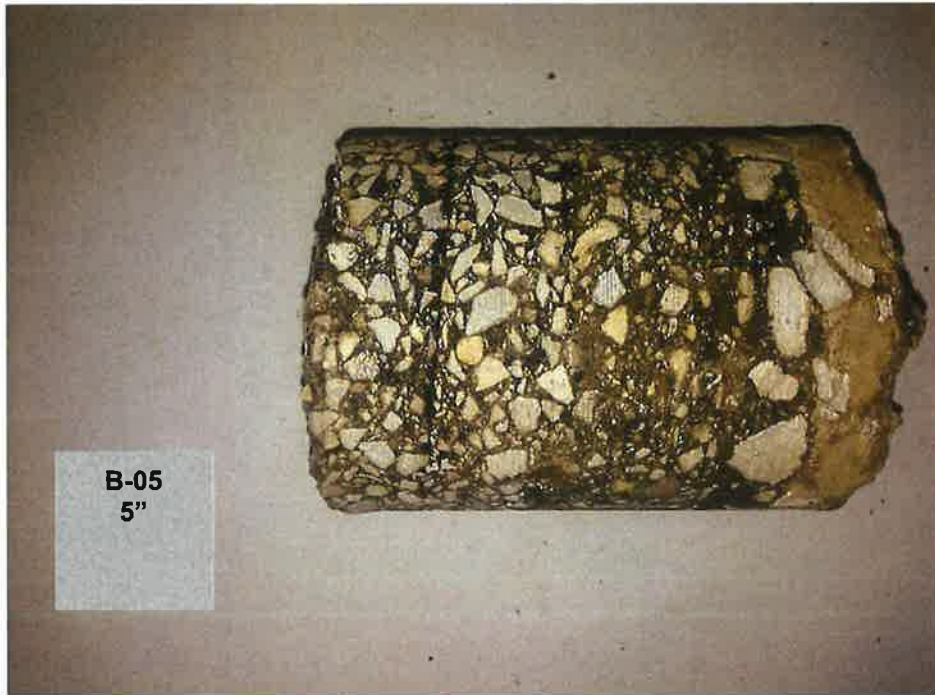
PHOTOGRAPH 19: Pavement core from B-05.
