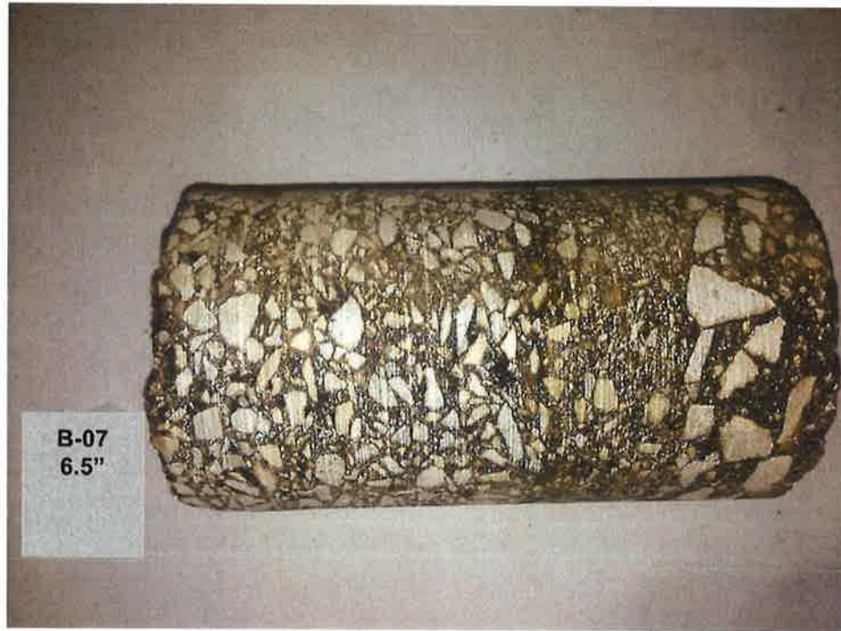
PHOTOGRAPH 21: Pavement core from B-07.
