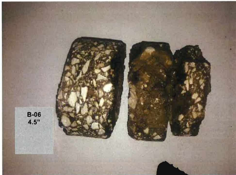
PHOTOGRAPH 20: Pavement core from B-06.
